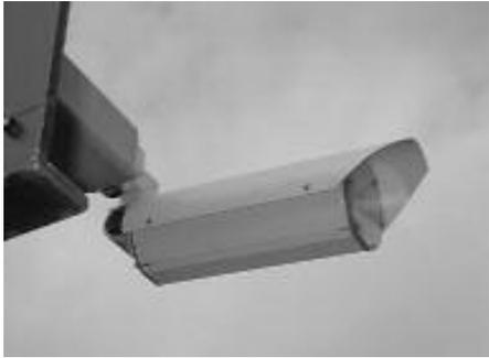
Camera on rail station (Alexandra Palace) ; part of a system to allow the train driver to see the whole platform
